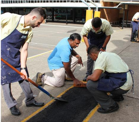
The students calculated the amount of concrete required, completed a safe work method statement, planned and organised all tools and equipment required. Thirty bags of pre-mix cement were hand mixed and placed in the formwork. The students worked as a team and every member contributed to the practical task.
