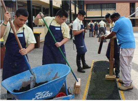
area of the school grounds and constructing a ramp. The students under the supervision of Mr Narayan, safely installed formwork, levelled trenches, reinforced, placed and finished concrete for the construction of a minor slab for a pathway and a ramp.
